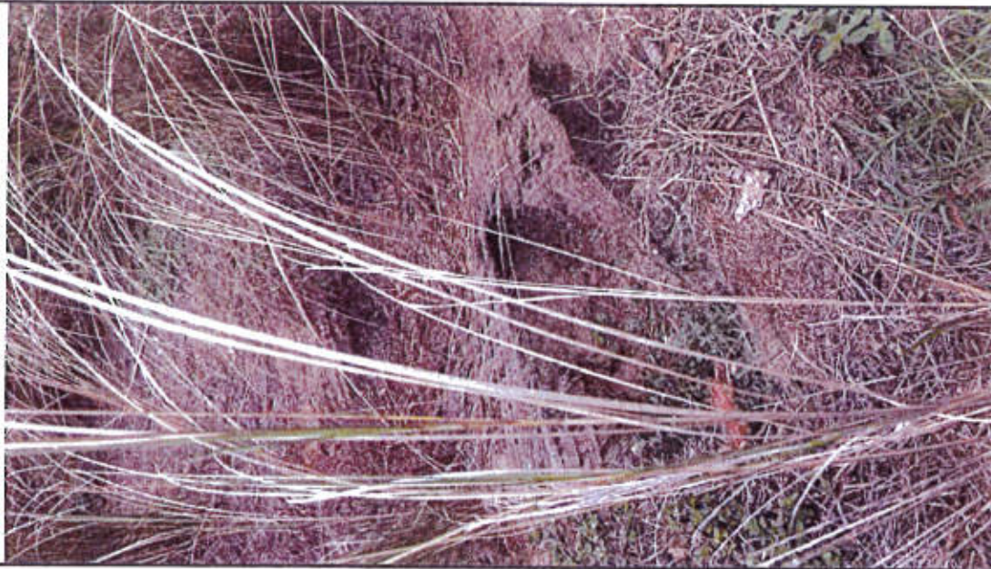
Photo 14: Slope erosion – northeast corner.
