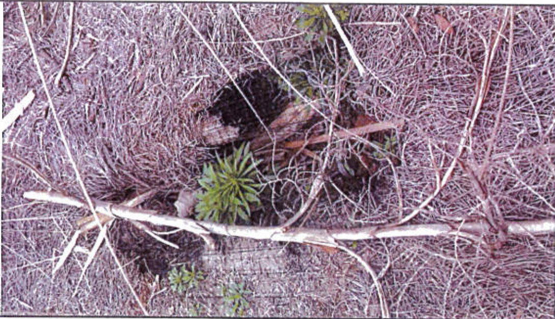
Photo 9: Slope erosion – northeast corner.
