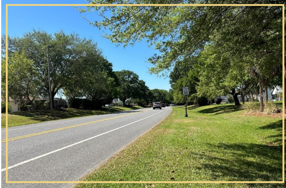
Photograph 1 - Morse Boulevard existing roadway conditions
