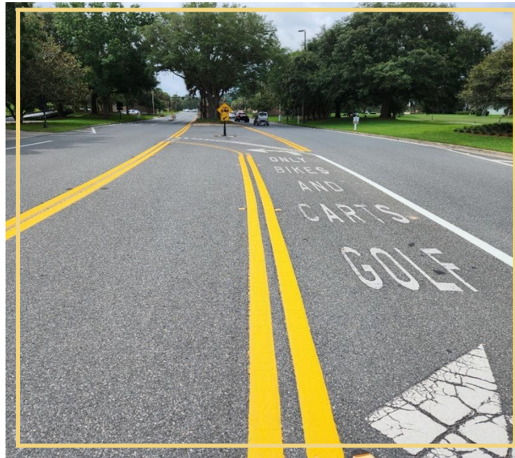
Photograph 6 - Marked golf cart crossing of Morse Boulevard at the C 466 gate
