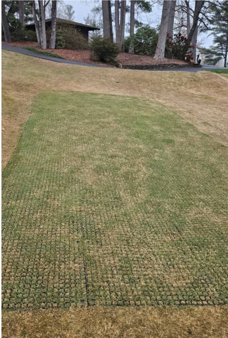
Figure 10: Traqmatz material was installed during the winter which protected the turf from excess traffic.
